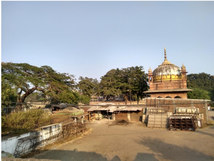
Figure 4.5 View from roof of Masjid
