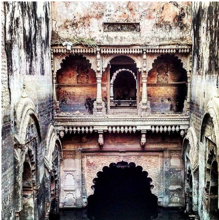
Figure 4.10 Entrance to baoli clogged with water
