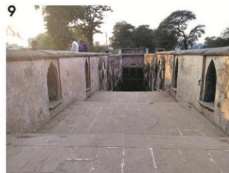
Entrance to stepped well
