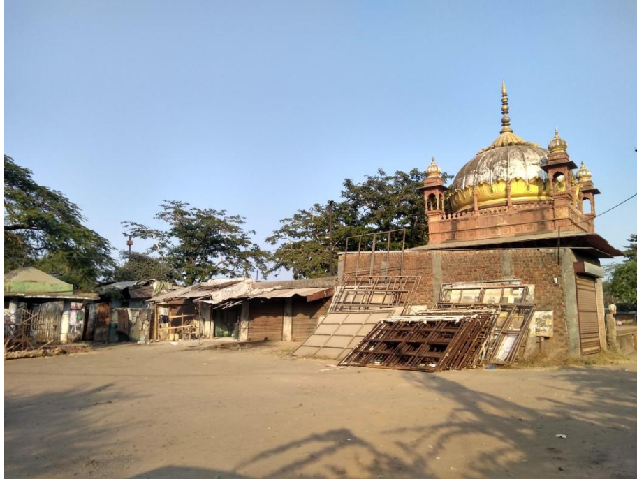
Figure 4.14 Encroachments around Nazar Mohammed Khan
