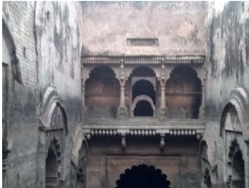
Figure 4.8 Ornamented Arched entrance to the baoli
