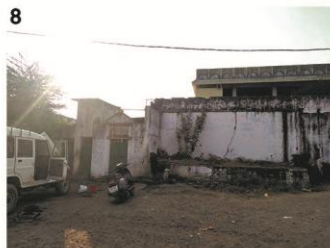
Encroachments along Masjid
