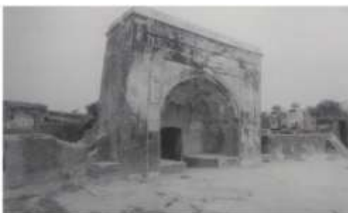
Figure 32 View of Sardkhana, Aam Khas Bagh
