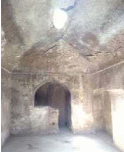
Figure 45 Image showing vault over a chamber of Hammam
