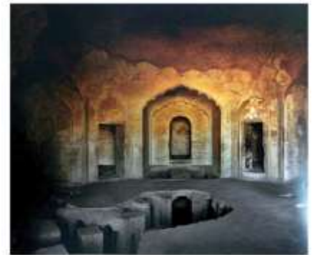
Figure 23 Interior of Shahi hammam, Agra fort Source: George Mitchell
