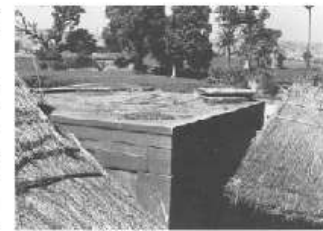
Figure 31 Cold Hammam of Dholpur with trabeated roof structure
