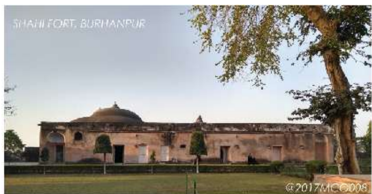
Figure 25 Shahi hammam, Burhanpur
