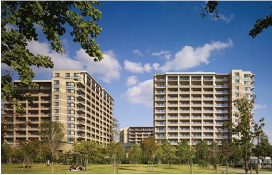
Figure 36. View of Tsukaguchi Senior Housing Community <BAR Architects>
