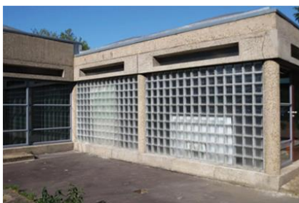
Figure 47. Clerestory Windows, Glass Bricks and Skylights to Allow Natural Lighting <Archdaily>
