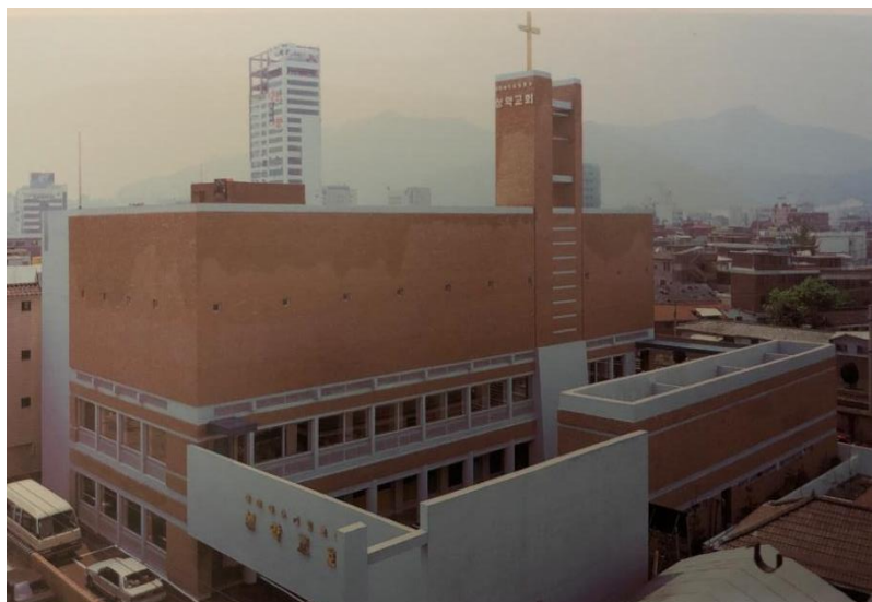
Figure 2.5: Presbyterian Church, UijeongBu, South Korea (Source: Modern Churches)
