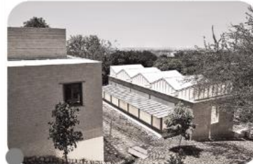
(Above) Visitor's Gallery Sawtooth gallery with marble sheet roofing for optimum level of natural lighting.
