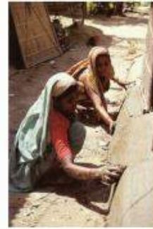
CONSTRUCTION OF PLINTH
