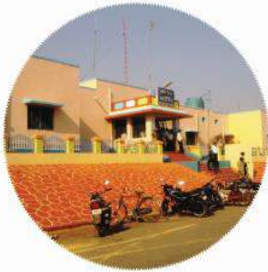
CONTAI RAILWAY STATION
