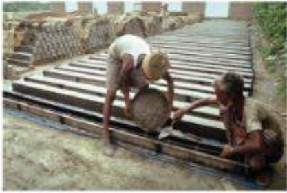
Laying of Plinth
