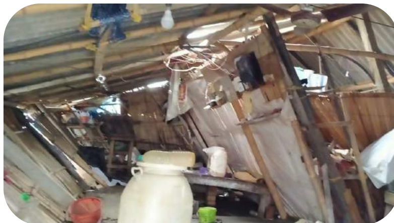
Figure 80 Collapsed Kuccha House (Source: Photo obtained from village
