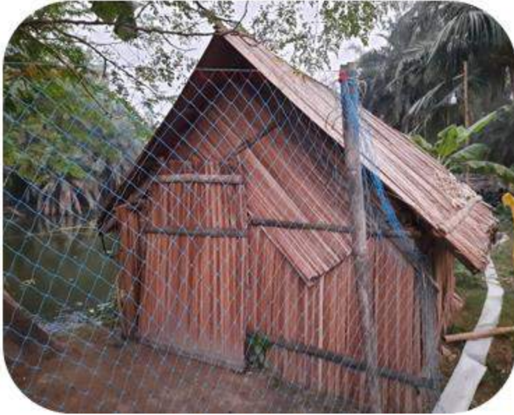
Figure 86 Image of Existing Shelters on the Site (Source: Author)
