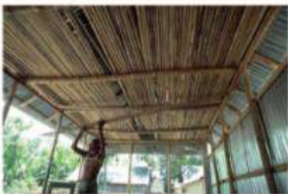
Reinforcing of Bamboo
