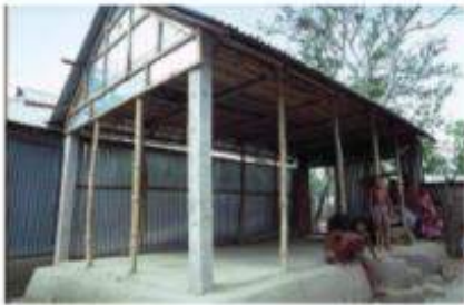
BASIC PLOT: CONCRETE SLAB FOUNDATION AND RCC COLUMNS
