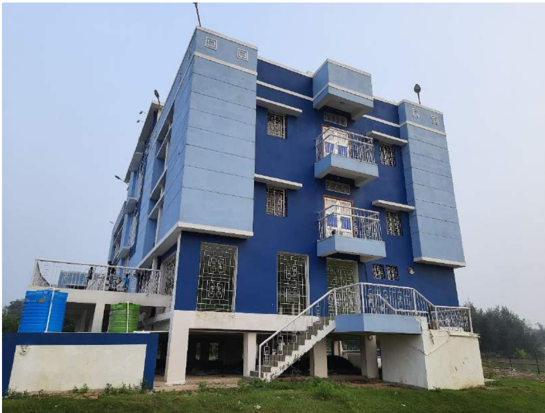
Figure 102 Existing Multipurpose Cyclone Shelter (Source: Author)
