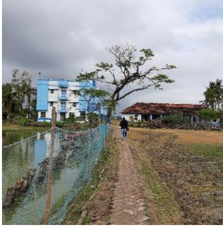
Figure 46 Bijoybati Multipurpose Cyclone Shelter (Source: Author)
