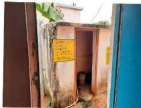
Figure 53 Images of ODRP Housing Units (Source: Author)
