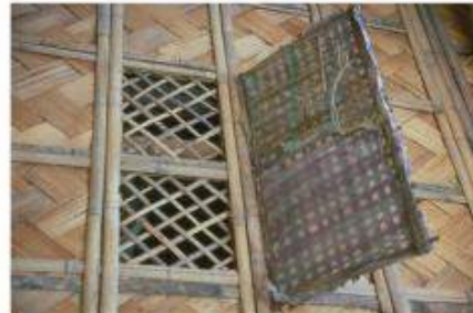
WINDOW WITH RUSH SIDING REINFORCED WITH BAMBOO
