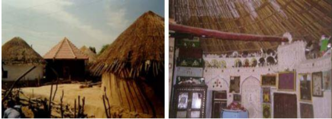
Figure 26: Left-Critical structural detail, Right- Interior view of house
