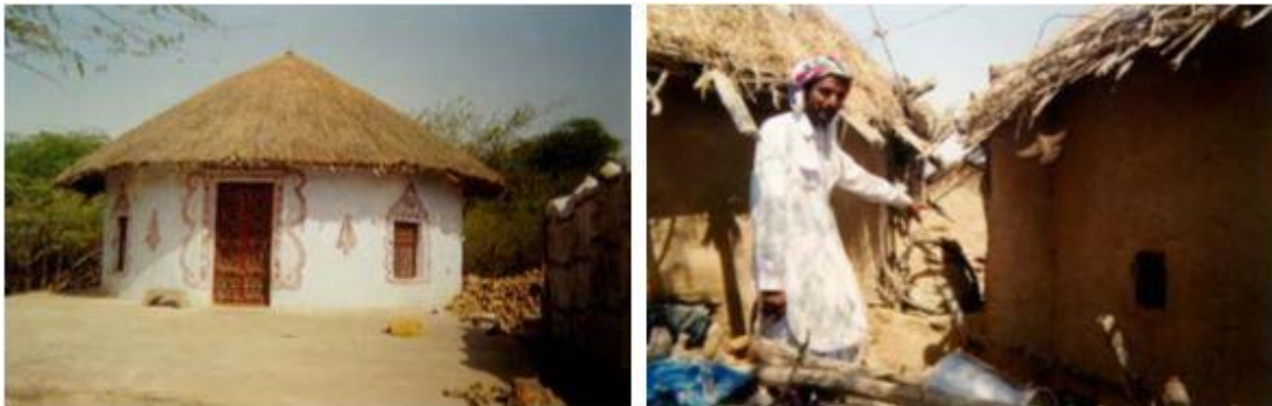
Figure 25: View of a single unit
