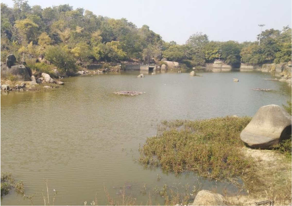
Figure 4.37: Images showing the degraded condition of Kola taal
