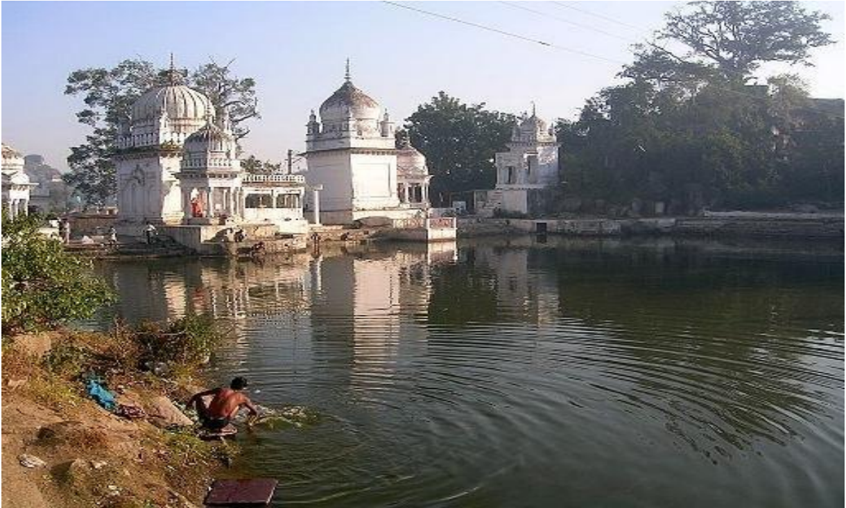
Figure 4.29: Images showing the degraded condition of Dev taal
