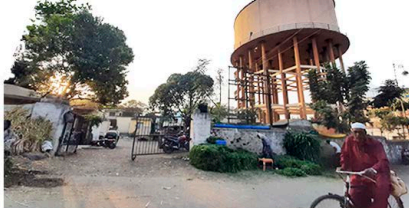
Water tank built in place of the Mandi
