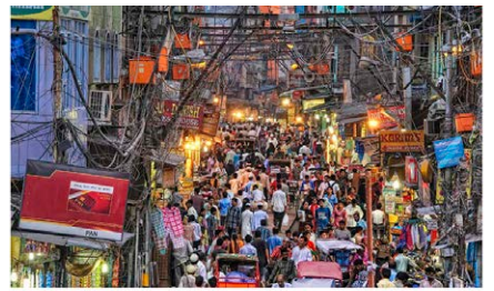
Cables and wires hanging from poles affecting the visibility of monuments and causing threat to the public
