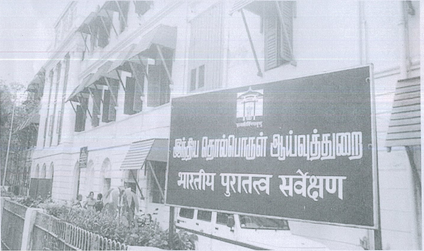
The building of the Department of Archaeology, Office of the Archaeological Survey of India. (File Photo | EPS)
