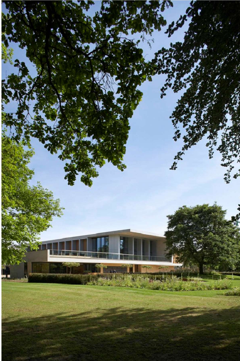
Fig. : 6.15 –Sainsbury Laboratory https://www.archdaily.com/154728/sainsbury-laboratory-stanton-williams
