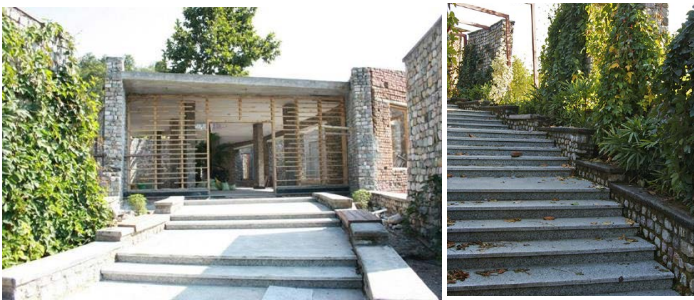
Figure Visitors Center Entry
