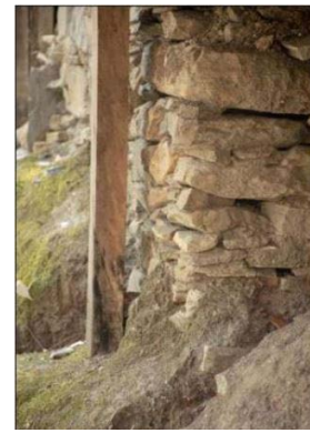
Figure 1-1.5-foot-deep random rubble masonry foundations to enable less soil erosion.
