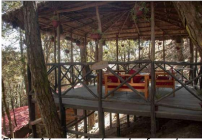
Figure A lounge deck made of wooden posts and thatched roof is provided for the users to
