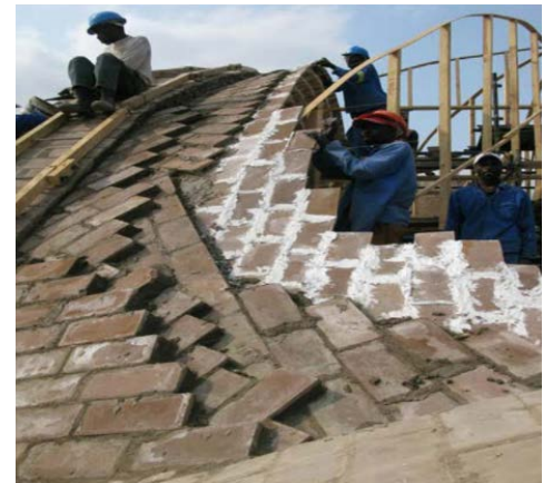
Figure Roof Construction
