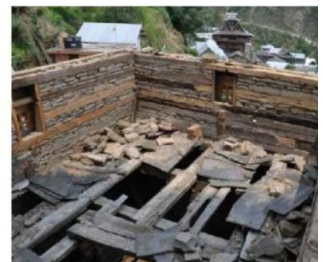
Figure 17 Laying of loose infill stone and wooden members.
