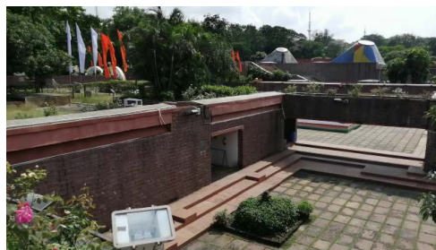
Figure Bridges connecting the
