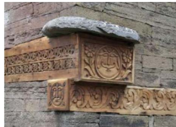
Figure 16 Ornamented Wooden Structural Members
