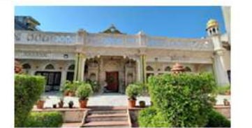
7. Residence of Rambabui
