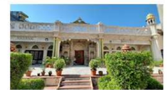
7. Residence of Rambabui
