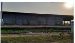
4. Storage space at railway line
