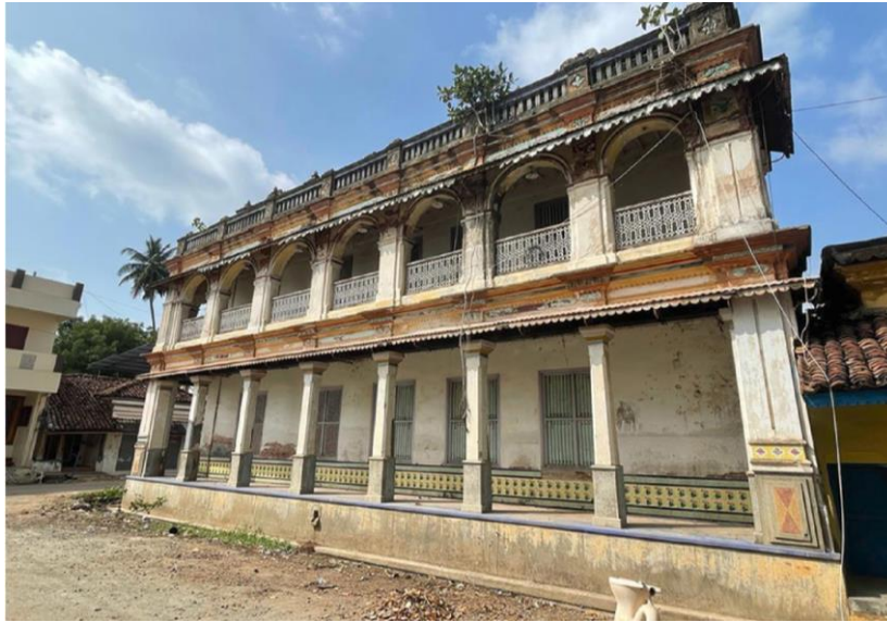
Fig.68. Franco-tamil style Mansion at Perumal Street
