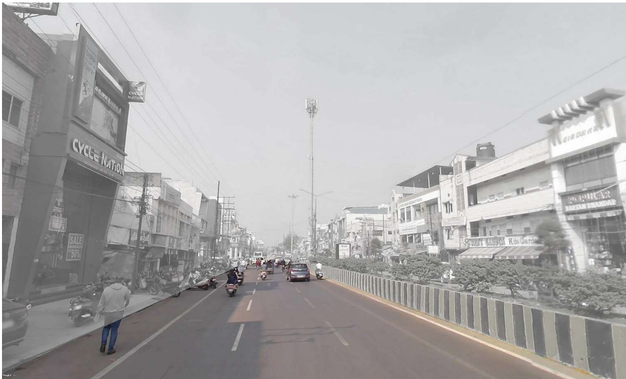
Figure 5 Pavement Quality of other major road of Indore
