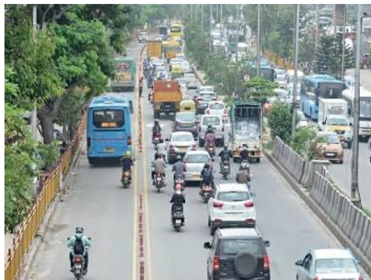
Figure 18 Kerb side lane BRTS corridor
