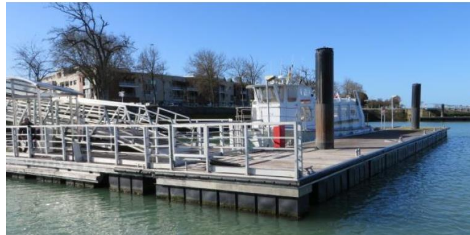
Floating pontoons to be covered with sheds
