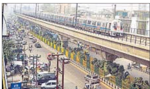
DMRC will develop 300 metres outside 15 upcoming stations to accommodate all types of vehicles.
