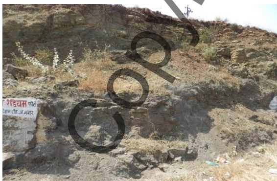
Figure 43 - Rock strata on road edge
