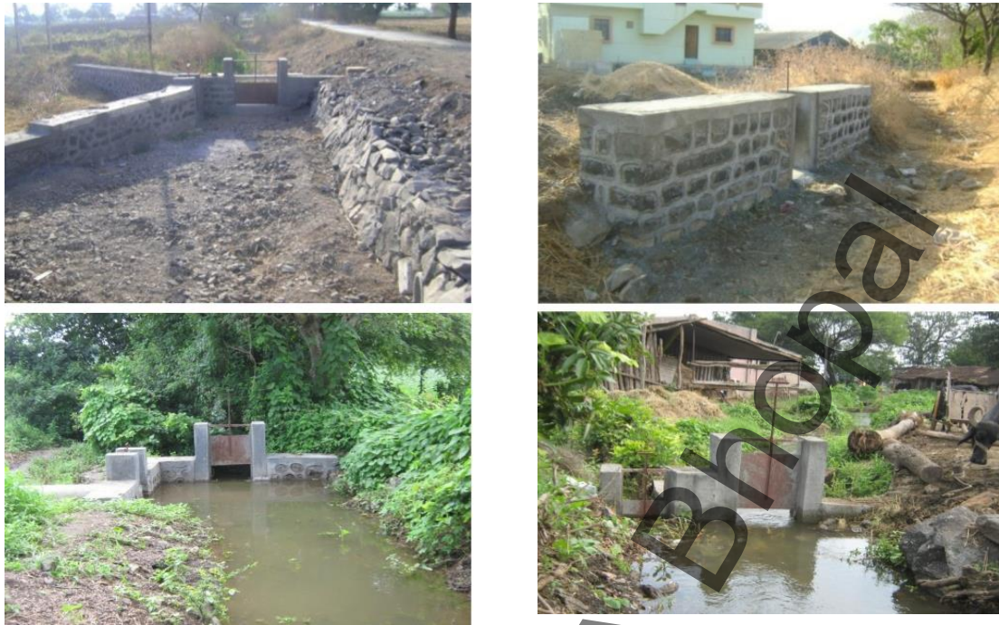
Figure 25 - Repairing work finished before monsoon
