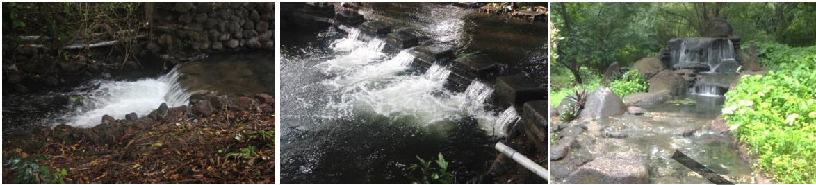
Fig. 58 Introducing levels in the stream for aeration
