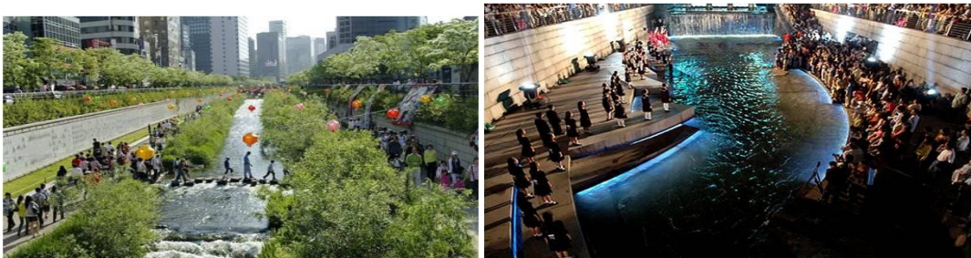
Figure 30. Condition of stream after restoration
