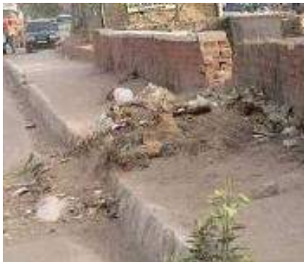
Figure 2.3/ 2.3: Uneven Surface due to lack of proper base that obstruct the walkway.
