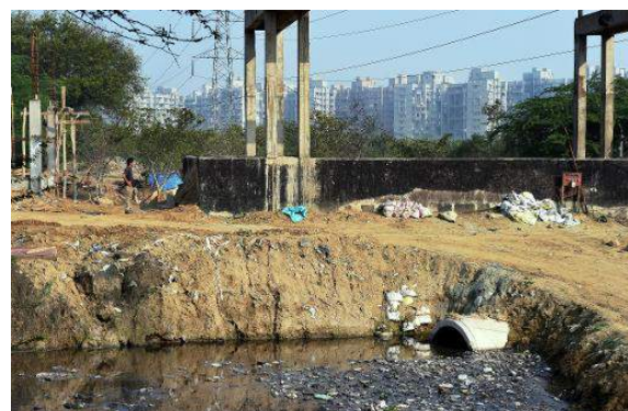
Figure 2.5: Unmanaged Water/ Sewage/ Storm-water Discharge.
