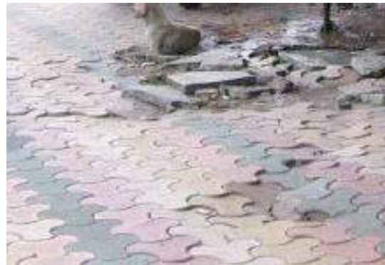
Figure 2.3/ 2.3: Uneven Surface due to lack of proper base that obstruct the walkway.
