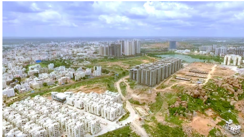
Figure 1-4 Urbanisation overburdening the city's landscape
