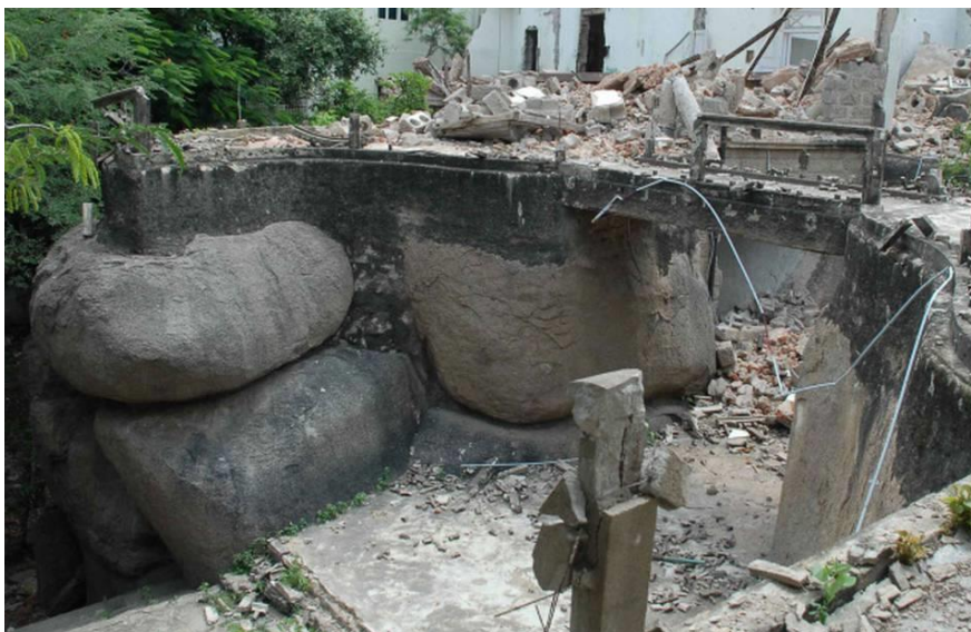
Figure 2-10 Recent photograph of Banjara Bhavan destroyed to make way for new development
