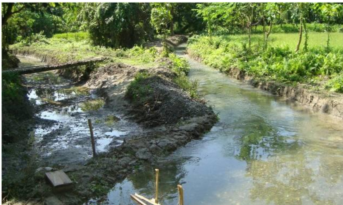
Figure 19: Dong water harvesting system
