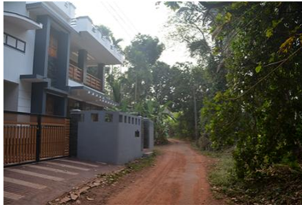
Figure 23 Encroachment on the sides of the road
