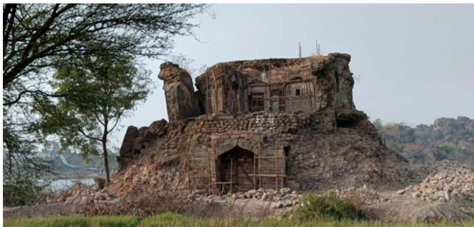
Figure 25 Ruined State of Monument
