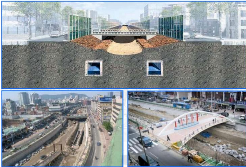
Stage 4: Sewer, road and bridge construction (September 2004)
