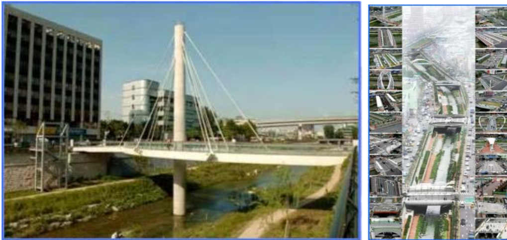
Figure 9. Bridge Construction (no.22)
