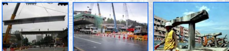
Stage 2: Highway demolition (August 2003)Stage
