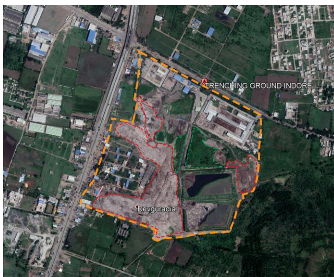
Figure 11. Indore trenching ground
