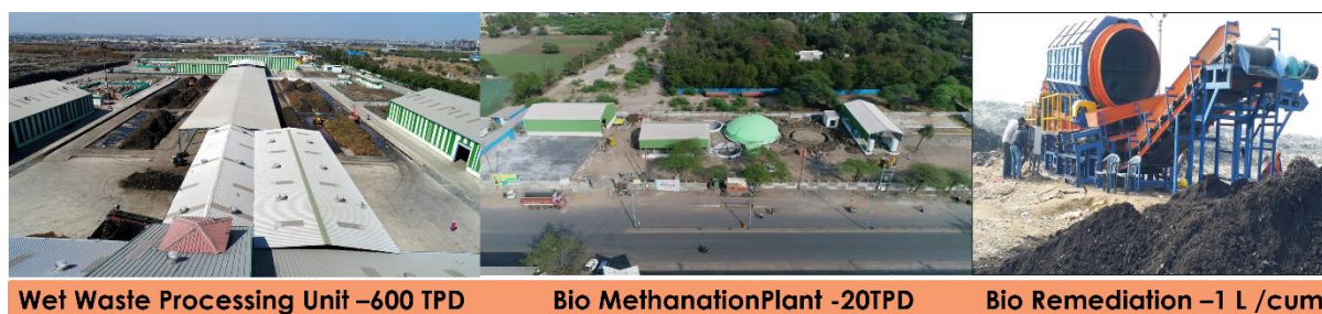
Figure 10. Indore trenching ground site pictures
