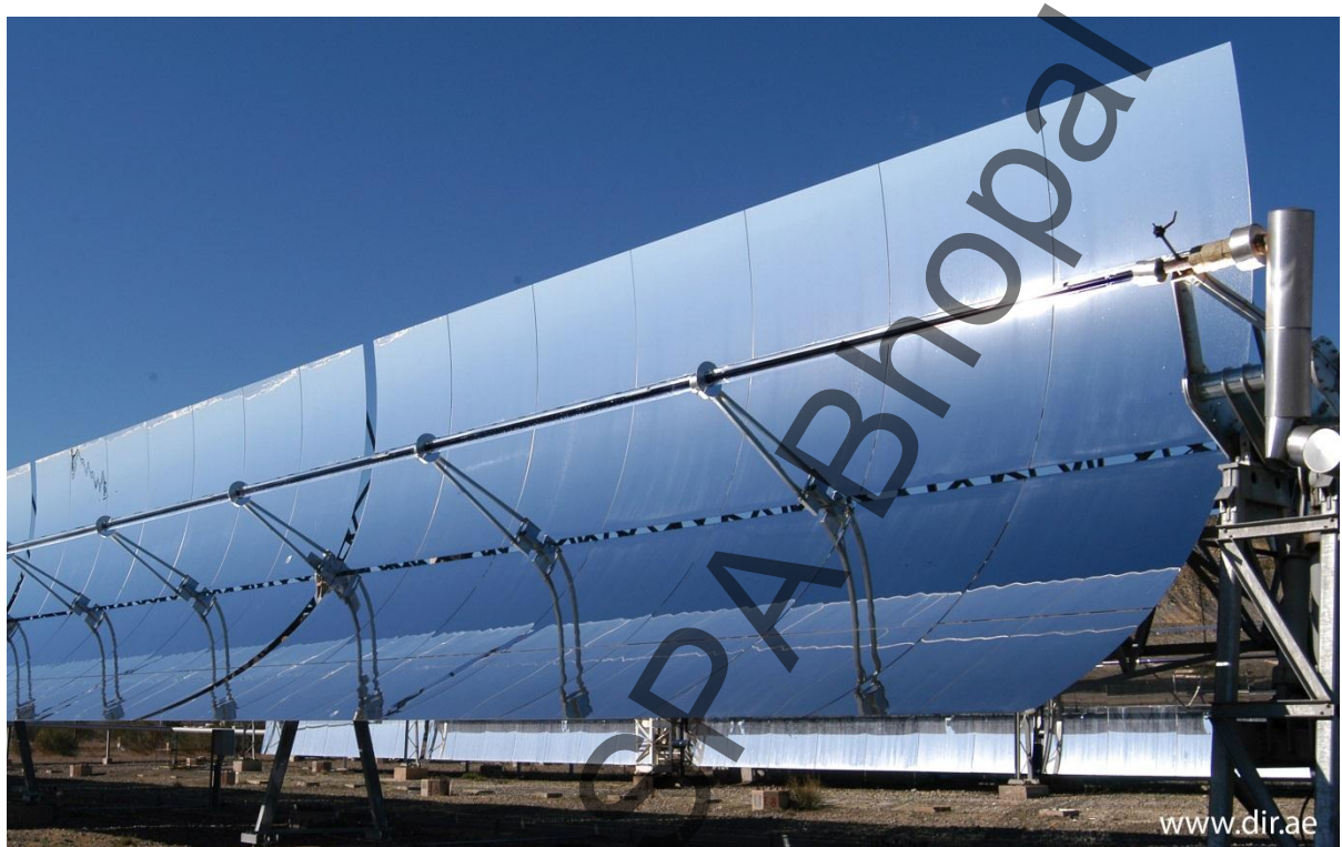
Figure 22: Concentrated Solar Power (Type 1)
