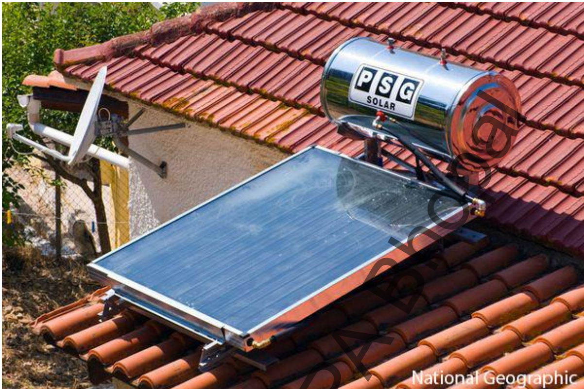
Figure 25: Solar water heater
