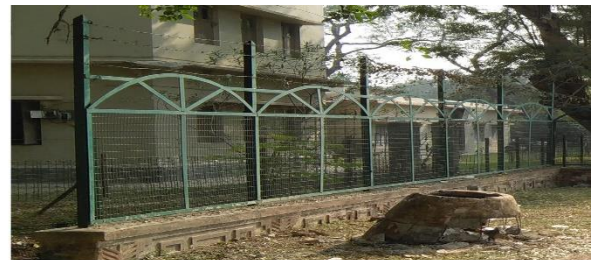
Fig: Internal Gate & Boundary wall
