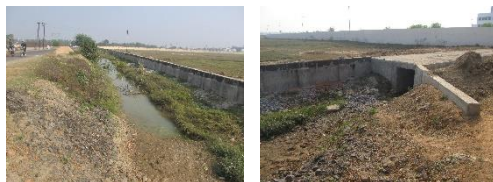
Open drain adjacent to the proposed
