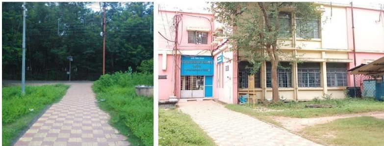
Fig: Concrete paver Pathway
