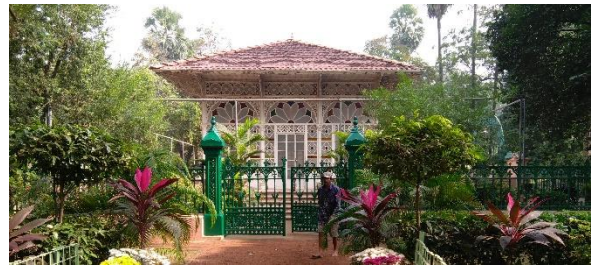
Temple (Upasana Griha)- green on both side enhancing the building
