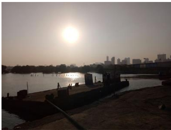
Figure 29 Jetty and Wharf at docks
