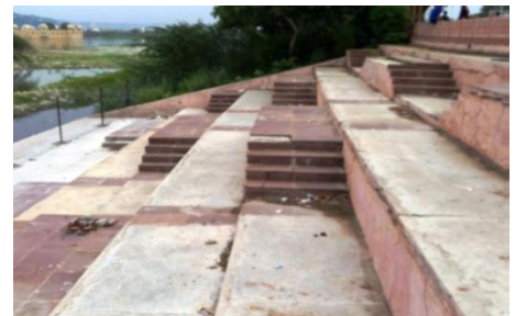
Figure 25: Constructed shoreline along lake Shoreline
