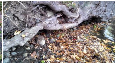
Figure 32: Exposed Tree Roots Being Undercut
