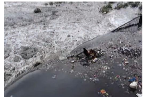
Figure 23: Sewage water Inflow in Mansagar Lake
