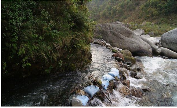
Fig.3.20. The kuhl (left) is diverted from the glacier-fed stream (right). SOURCE: (indiawaterportal August 2014)
