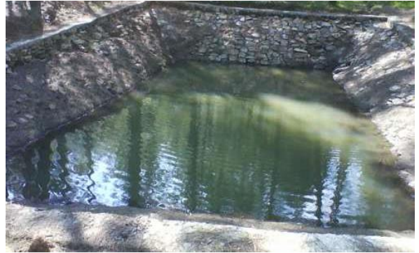
Fig.3.23. Stone pitched pond, SOURCE: (www.gramya.in August, 2013)
