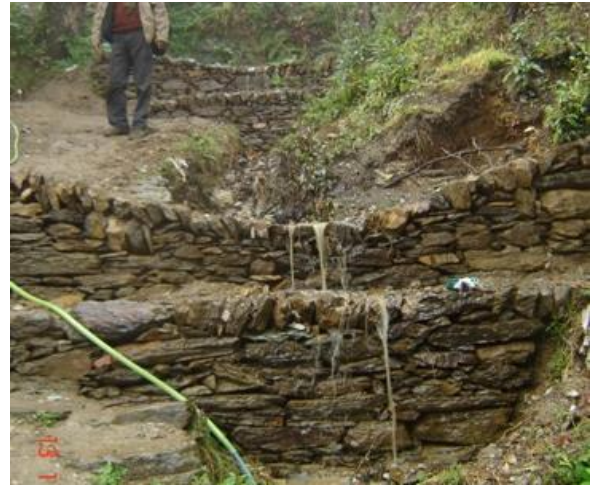
Fig.3.25. Dry stone check dams, SOURCE: (www.gramya.in August, 2013)
