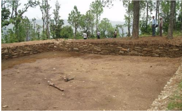
Fig.3.22. Dry stone check dam, Silalekh SOURCE: (www.gramya.in August, 2013)
