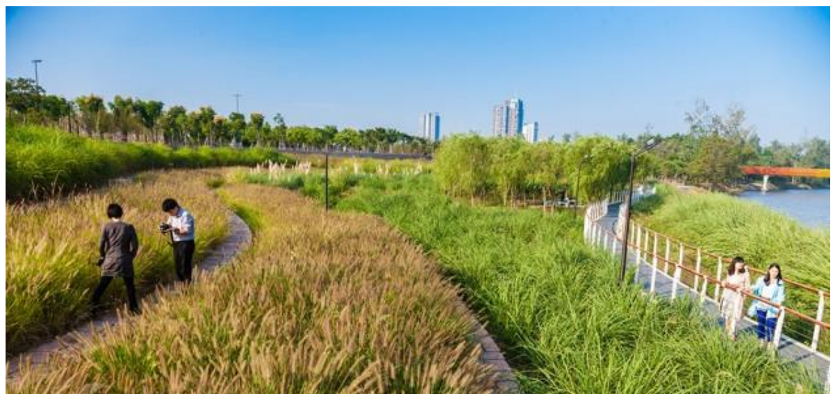
Fig.3.11. The beautiful terraced embankment was built by removing the concrete floodwall and through a cut-and-fill strategy that balances the earthwork on-site. The terraces create a flood resilient zone that allows people to enjoy the lush tall grasses adaptive to the seasonal floods.
