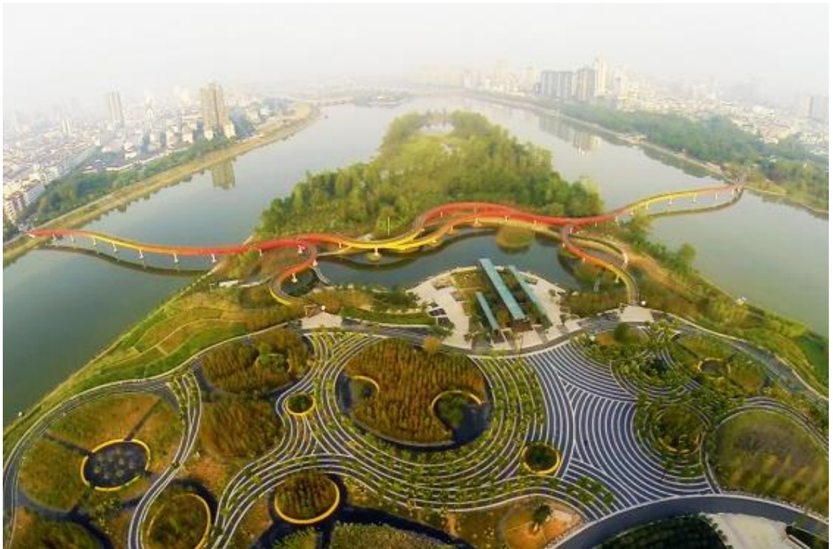
Fig.3.9. An aerial view of the park during the dry season, note the lush tall grasses covering the terraces on the embankment. The terraces are enriched by silt deposited during the flood season (view is toward the west, photo: November, 2014).
