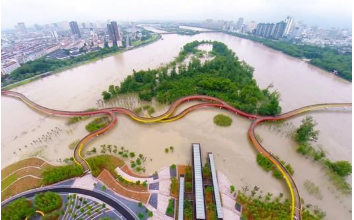
Fig.3.8. An aerial view of the park during the monsoon season showing a 20-year flood and testifying to the flood resilient design. Note the uninterrupted connection of the city through the bridge (the view is toward the west, photo: May, 2014).
