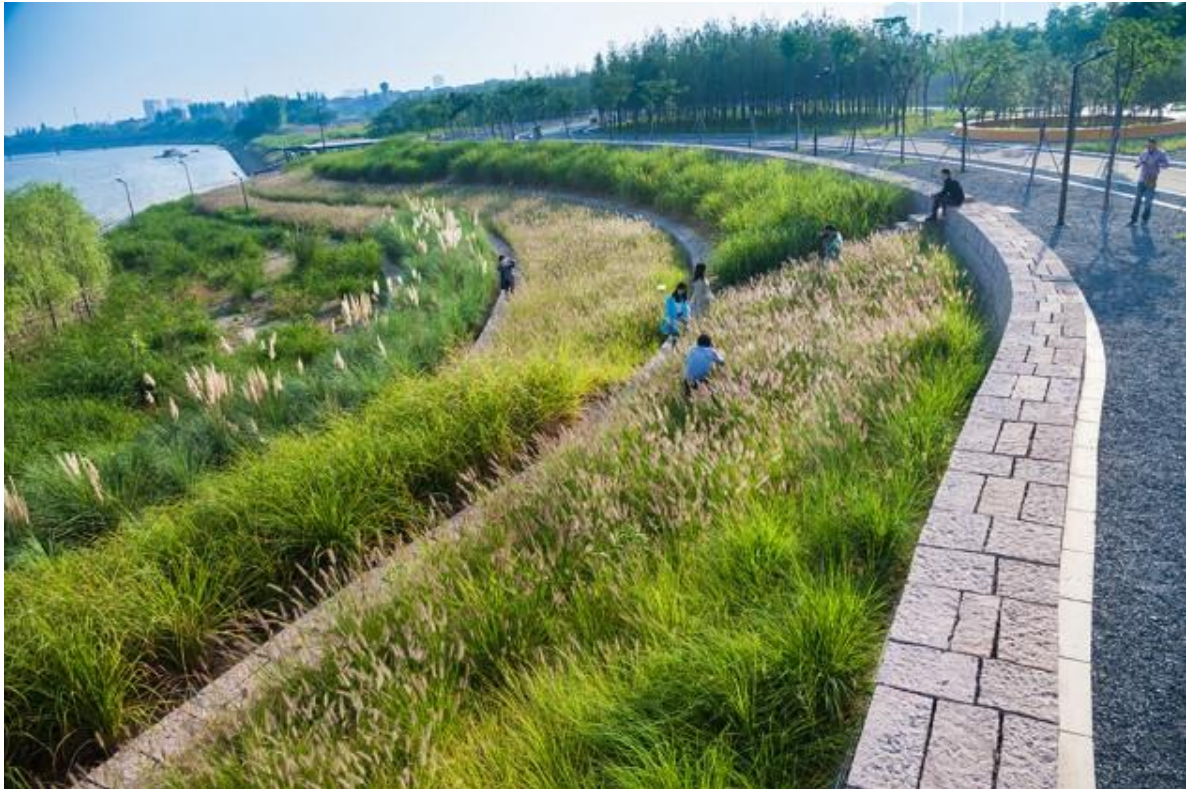
Fig..3.12. The terraced embankment in flood resilient zone is accessible through stairs and paths along the top of terrace walls for emersion within the varied texture, color and movement of the lovely grass panels (view is toward the east).
