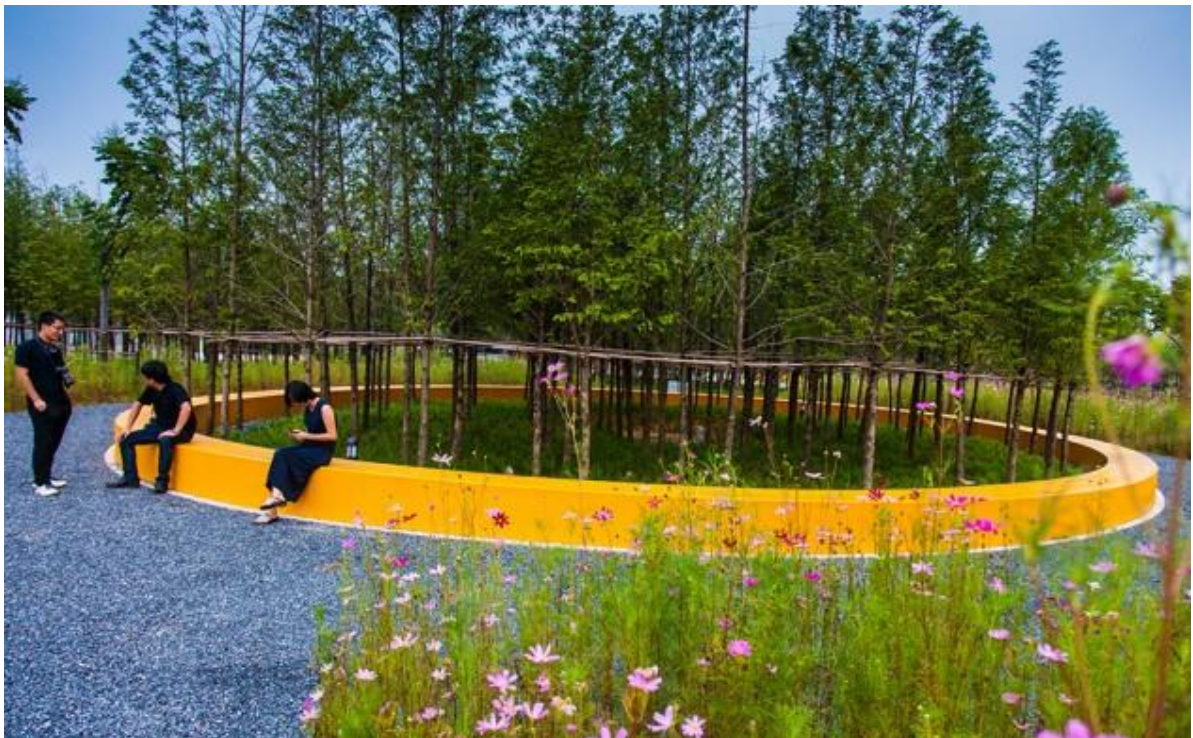
Fig.3.17. Circular bioswale. The surfaces include gravel surface bioswales for planting, and permeable concrete for automobile use.
