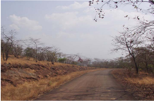
Figure 95: Soil erosion on the slopes
