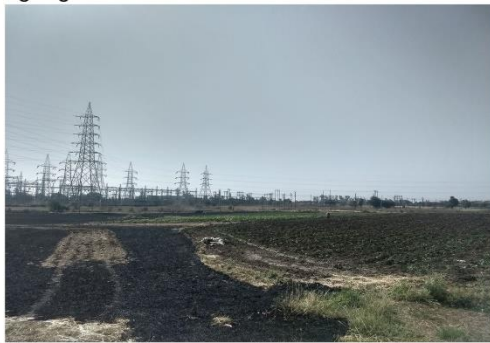
Wide view of the power station amidst the farms
