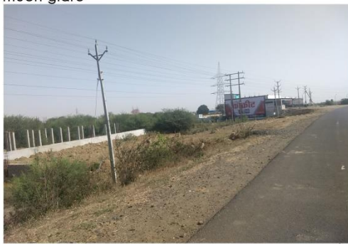
Edges are eroded, no trees, water contamination
