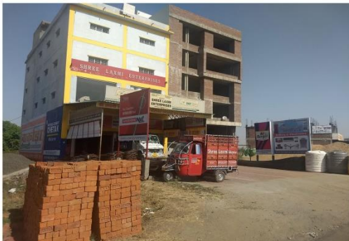
Encroached built structures, edge conditions
