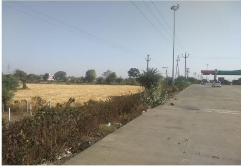
The eroded and unmaintained edges - toll plaza
