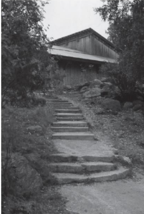
A more recent example from Germany uses natural stone, gravel and weathered rough sawn timber, which work together and fit their surroundings. Simplicity and good attention to the detail of construction make this a timeless solution.
