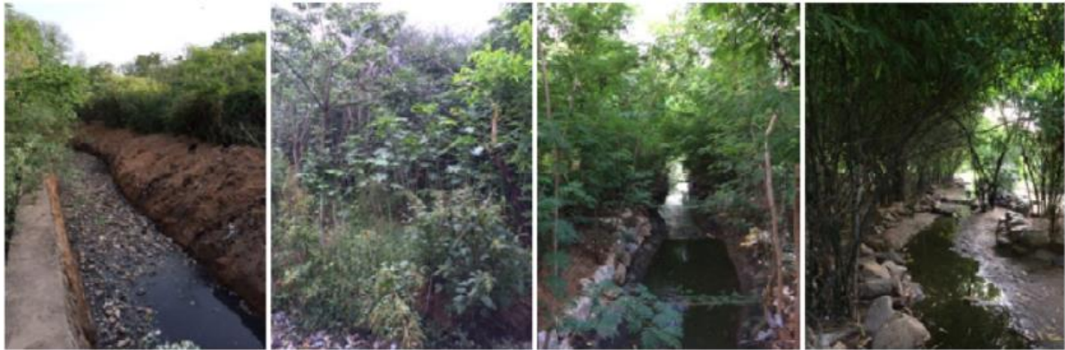
Figure 44: Greening of storm water drain banks as a phytoremediation and beautification strategy.
