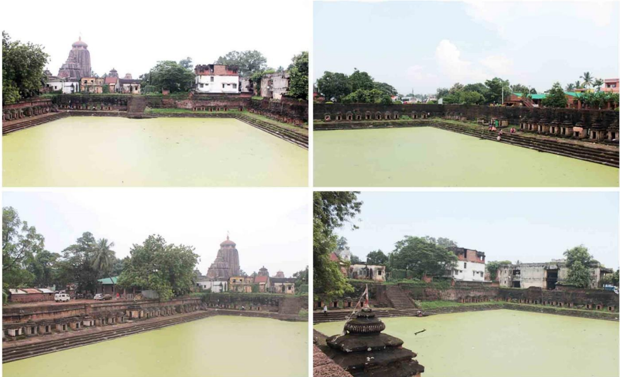
Figure 25: Devi Padahara tank
